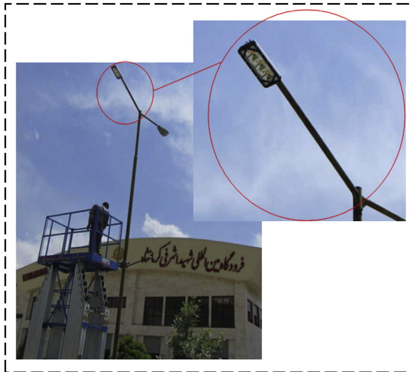
Fig. 1. A photo of the installed LED light in the airport of Kermanshah city, including the zoon of headlight for AWS.
