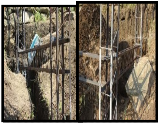
Figure 3.12 Modified Beam and Column's Reinforcement Connection
