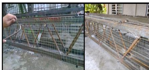
Figure 2.9 Actual Placement of Mesh
