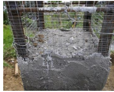
Figure 3.14 The Final Output of the Column using Ferrocement Formwork System
