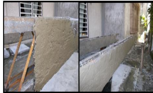
Figure 2.10 Actual Application of Mortar
