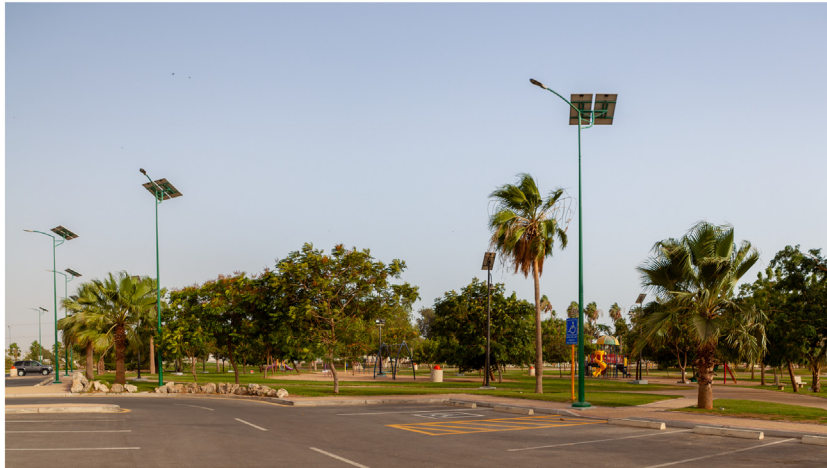
Fig. 5. A park in Yanbu with solar-powered lamp posts.
