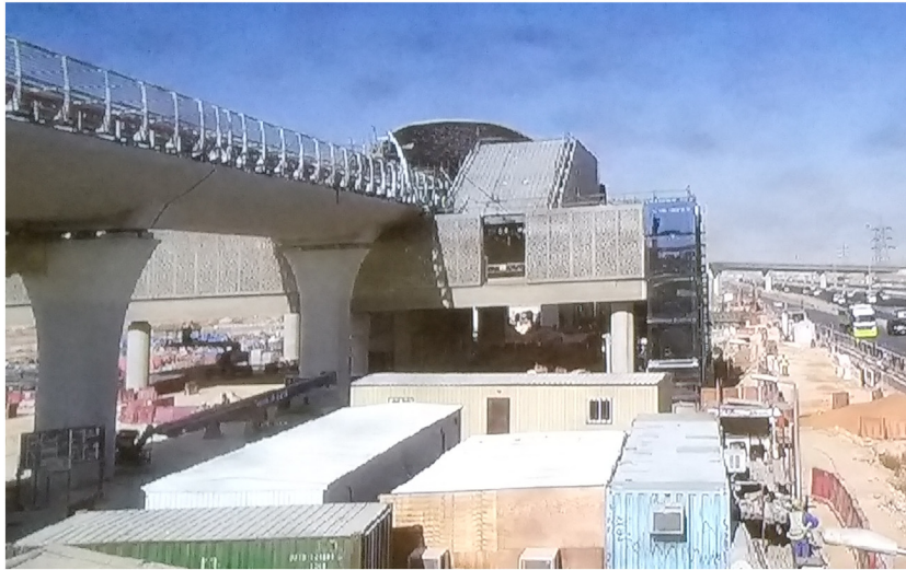
Fig. 4. Riyadh Metro line and station under construction.
