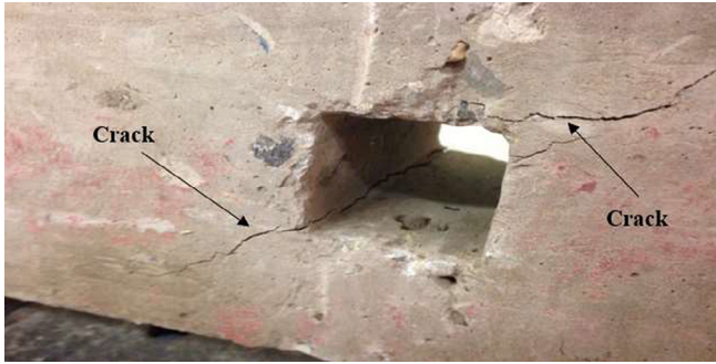
Fig. 3. Diagonal cracks around opening.
