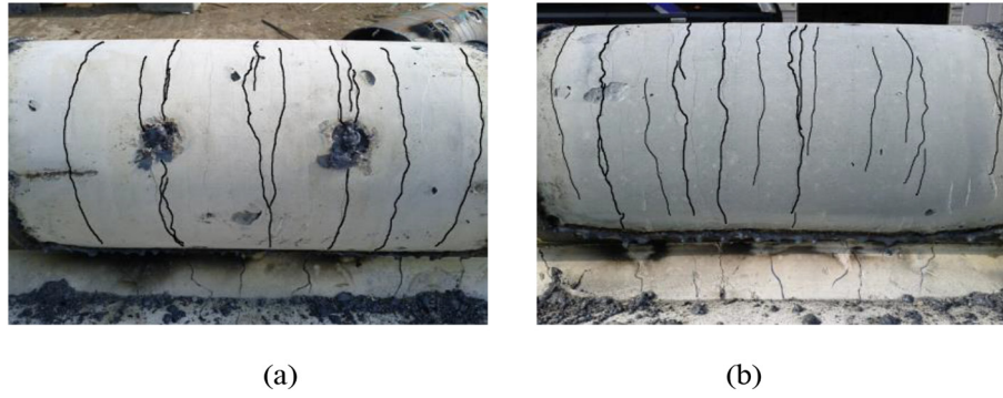
Fig. 10. Crack pattern of the concrete infill: (a) SC-P specimen; and (b) FC-P specimen.
