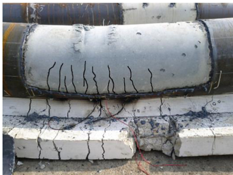
Fig. 15. Crack pattern of the concrete infill of the FC-N specimen.
