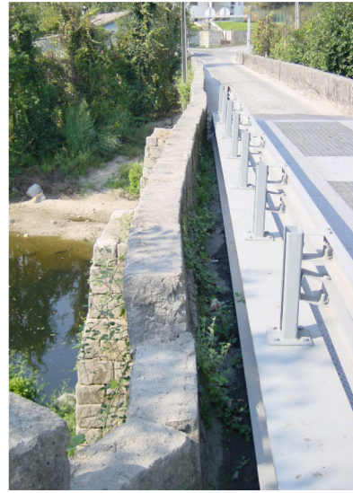
b) Out-of-plane deflection of the spandrel wall.
