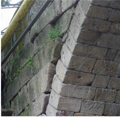
a) Sliding of the spandrel wall over the arch barrel.
