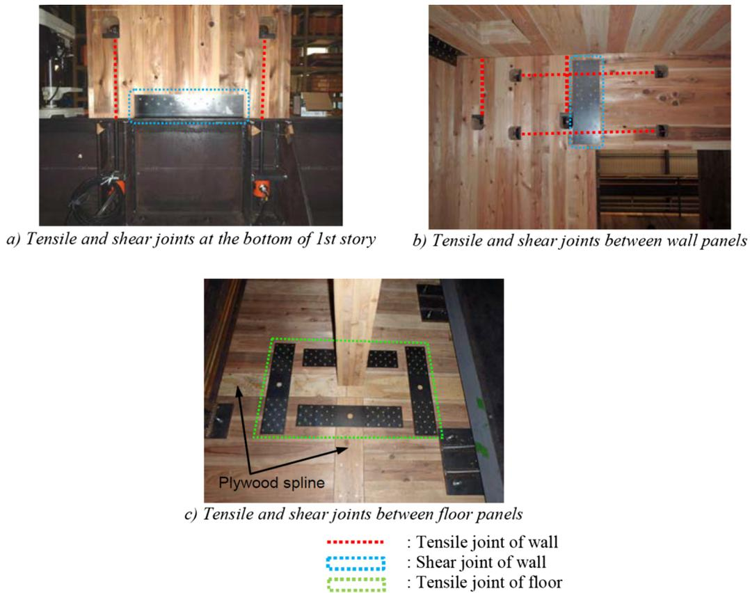
Fig. 8. Photos of connections.
