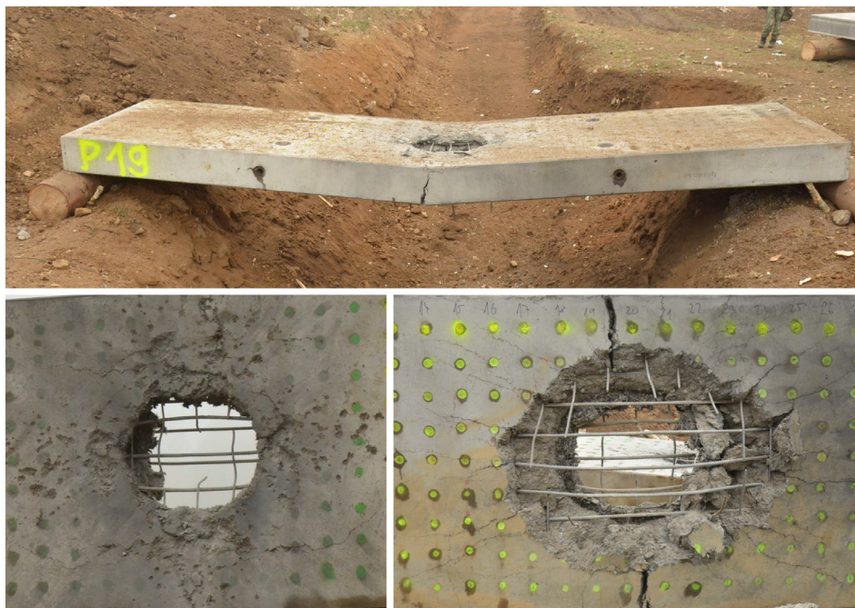
Fig. 7. Damage to specimen No. 19 after the blast. Overall view (top), top view (left), bottom view (right).
