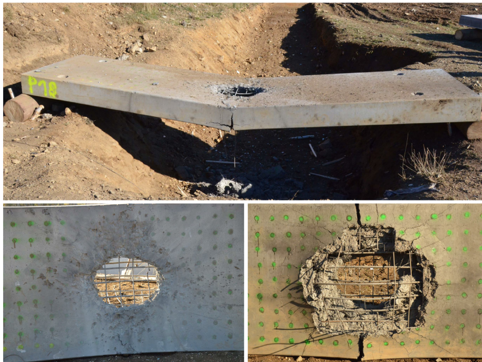
Fig. 6. Damage to specimen No. 18 after the blast. Overall view (top), top view (left), bottom view (right).
