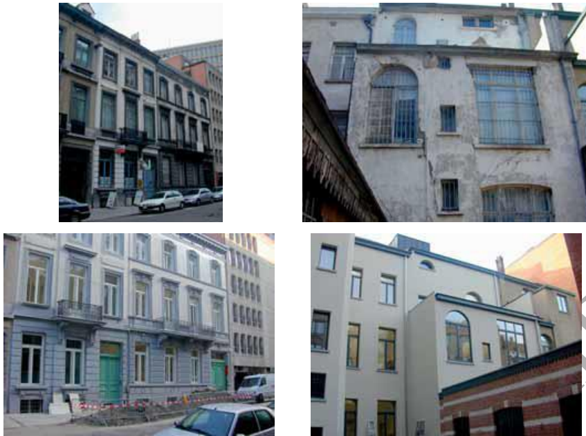
Figure 14. Renewable Energy House, Brussels (Belgium). Front and back facade (a) before refurbishment, and (b) after refurbishment [6].
