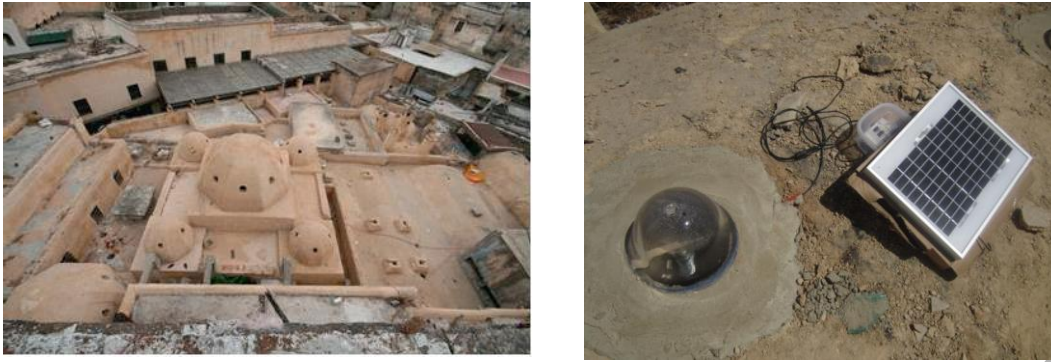
Figure 20. Hammam Seffarine in Fez (Morocco) and the solar lighting system installed [61].
