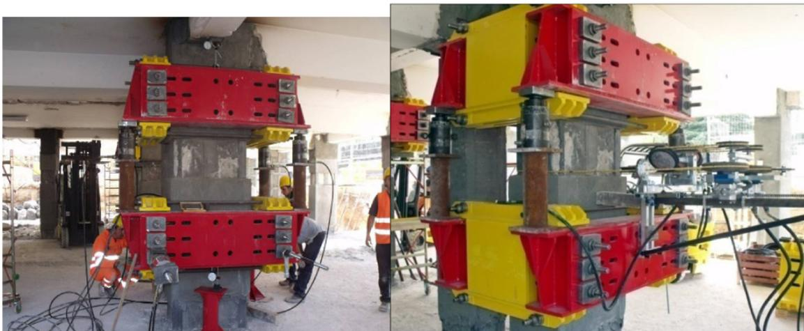
Fig. 16. Jacking, diamond wire cutting and extraction of the column block.
