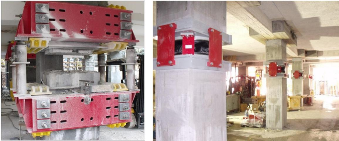
Fig. 17. Installation of the isolation units (locked) at the top of first basement columns.
