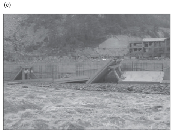
Fig. 14. Gaoshu Bridge during the 2008 Wenchuan earthquake: (a) elevation and plan views of original bridge (unit: m); (b) map showing bridge crossed by surface fault rupture; (c) collapsed bridge (Fig. 14a is generated based on information provided by Hui [53]; Fig. 14b is modified from Hui [53]; Fig. 14c is reprinted from Zhao and Taucer [149]).
