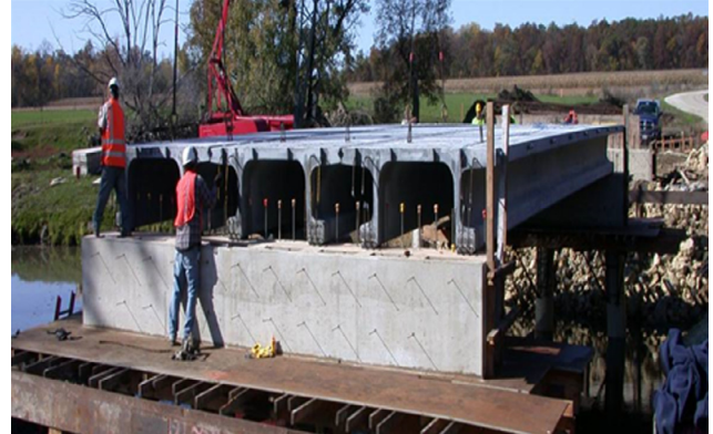
Fig. 4. American Jakway Park Bridge. (Source: www.ductal.com).
