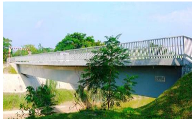
Fig. 8. Kampung Linsum Bridge. (source: Voo, Y.L. and Foster, S.J., "Malaysia First UHPC Prestressed Motorway Bridge", 2008).
