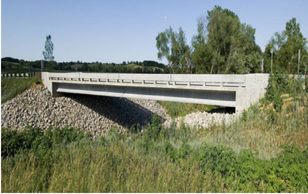
Fig. 2. American Mars Hill Bridge. (Source: www.ductal.com).
