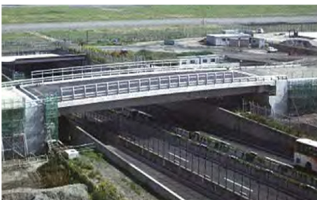
Fig. 7. Japan GSE Bridge. (source: Koichi Maekawa, "Designing & Building With UHPFRC Chapter 12", 2011).
