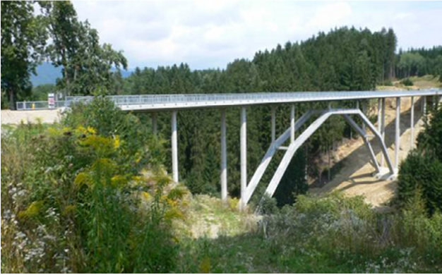
Fig. 6. Wild Bridge. (source: Nguyen, K., et al. "Assessment of serviceability limit state of vibrations in the UHPFRC-Wild bridge through an updated FEM using vehicle-bridge interaction", 2015).
