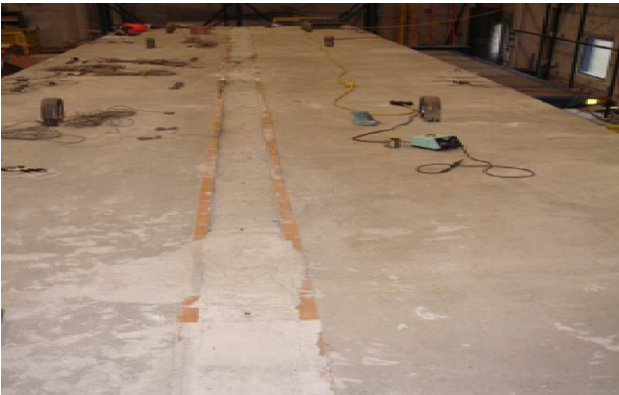
Fig.14. UHPC Connection of Two Girders.
