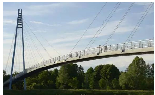
Fig. 9. Celakovice Pedestrian Bridge. (source: Koukolík P et al. "Construction of the First Footbridge Made of UHPC in the Czech Republic", 2015).
