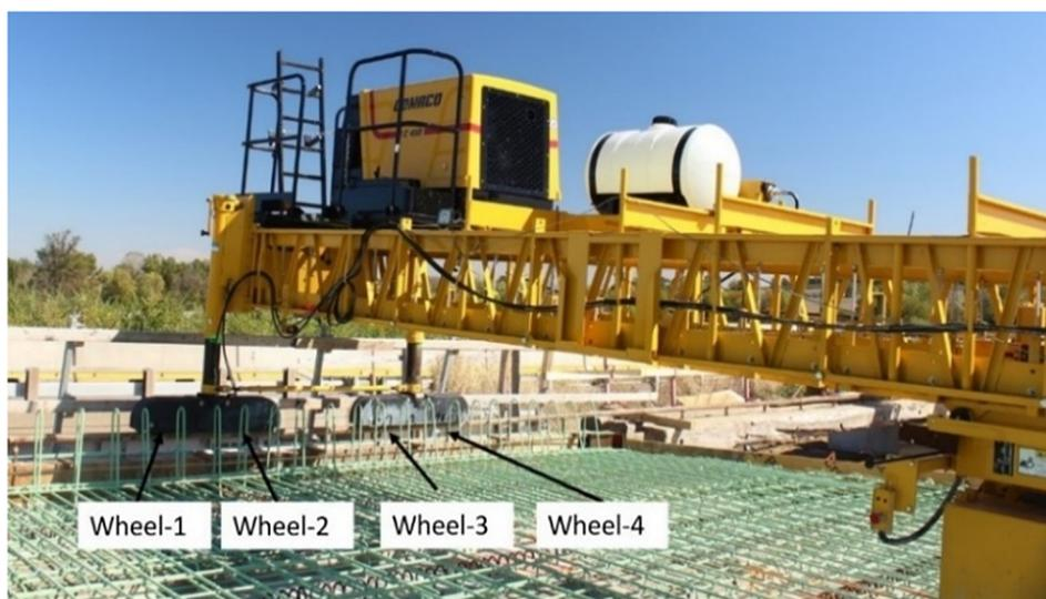
Fig. 3. Screed machine wheel load.
