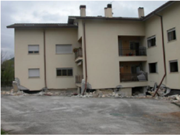
Fig. 1. Soft story failure [5]
