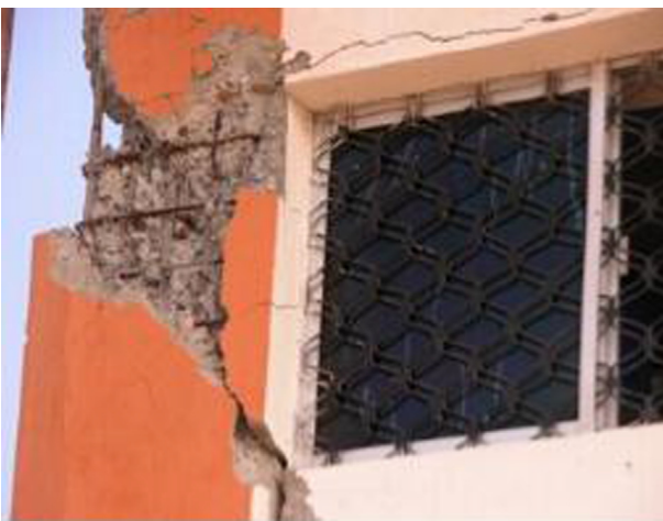
Fig. 2. Shear failure of short column [6]
