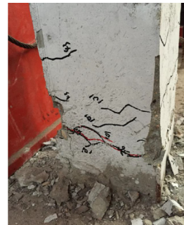
(c) crushing of column foot
