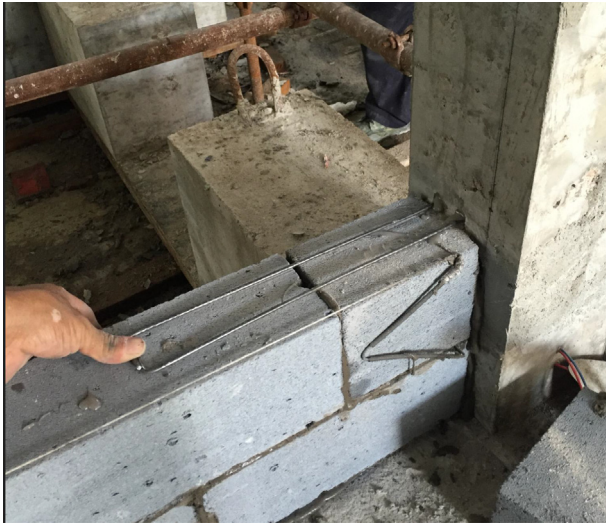
Fig. 4. Connect bars of infills.
