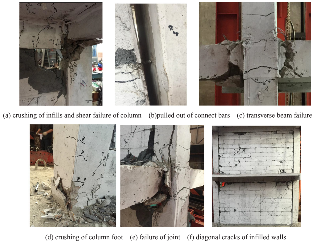
Fig. 9. Cracks of MRC-1.
