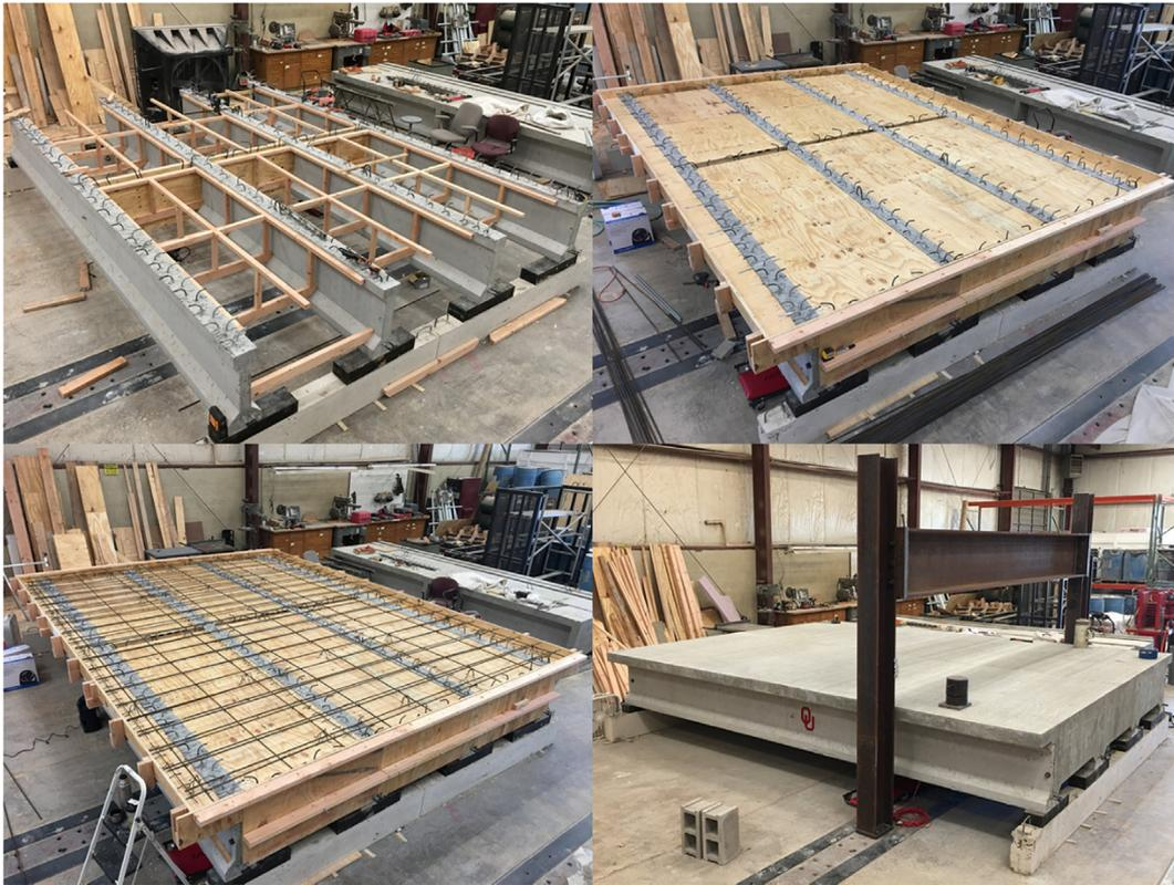
Fig. 3. Bridge construction progress. Top left shows girders laid out and beginning of formwork construction. Top right shows completed formwork including diaphragms. Bottom left shows deck steel. Bottom right shows completed bridge with load frame.
