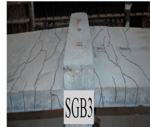
(d) cracks near middle support
