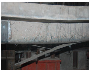
(b) peeling off of CFRP at left mid-span
