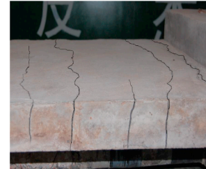
(d) cracks near middle support
