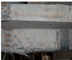
(b) tensile rupture of CFRP at left mid-span
