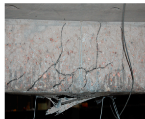
(c) tensile rupture of CFRP at right mid-span
