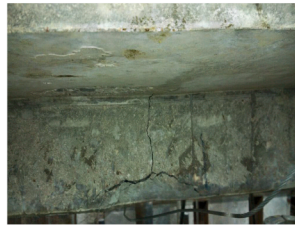
(c) horizontal crack at left mid-span
