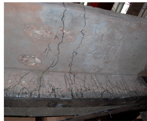
(c) cracks at the mid-span
