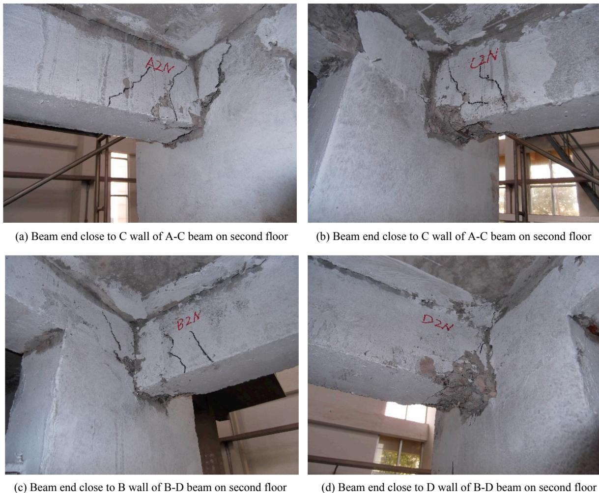
Fig. 25. Damage of second floor superposed connecting beams.
