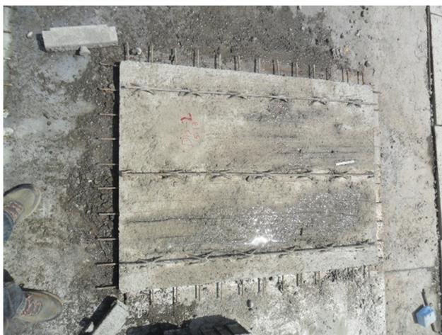
Fig. 14. Manufacturing of superposed floor slab.
