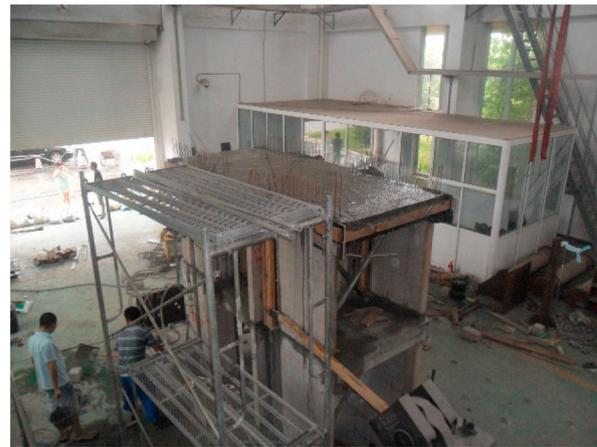
d. Concrete pouring for superposed components of second floor
