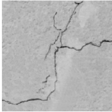
Fig. 2. Crack image of the concrete bridge
