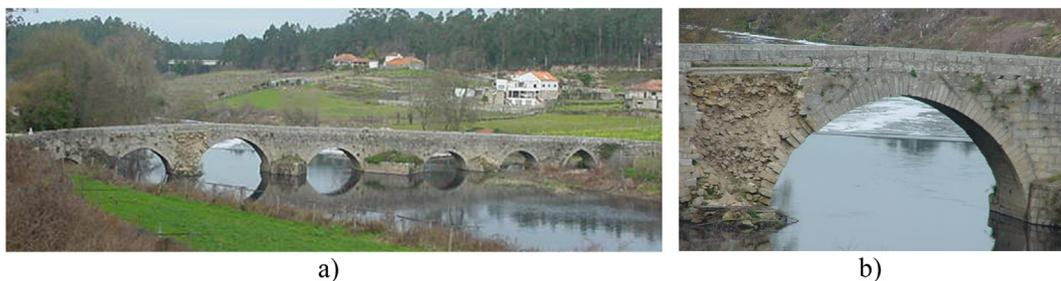
Fig. 2. D. Zameiro bridge: a) general view, b) partially collapsed pier.
