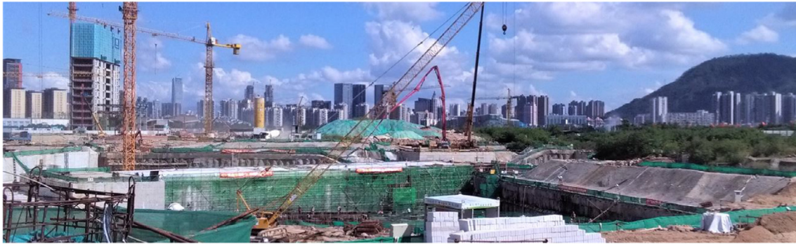
Fig. 1. A photograph of the Qianhai Tunnel under construction in Shenzhen.
