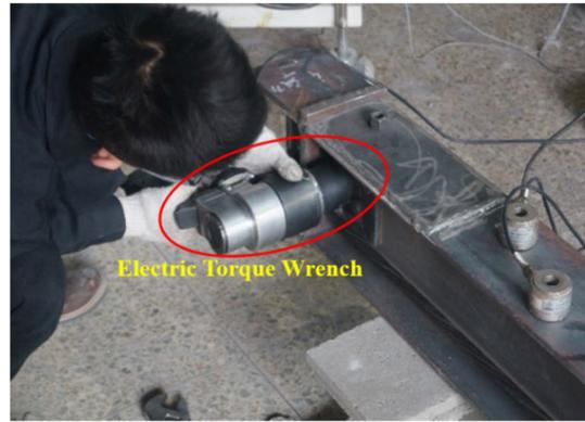
**Fig. 11.** Final screwing of high-strength bolts.
