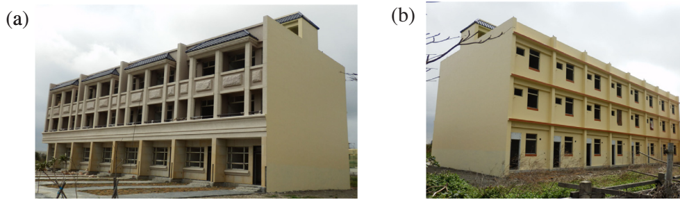
Fig. 1. Low-rise reinforced concrete row houses in Taiwan: (a) front view and (b) back view.
