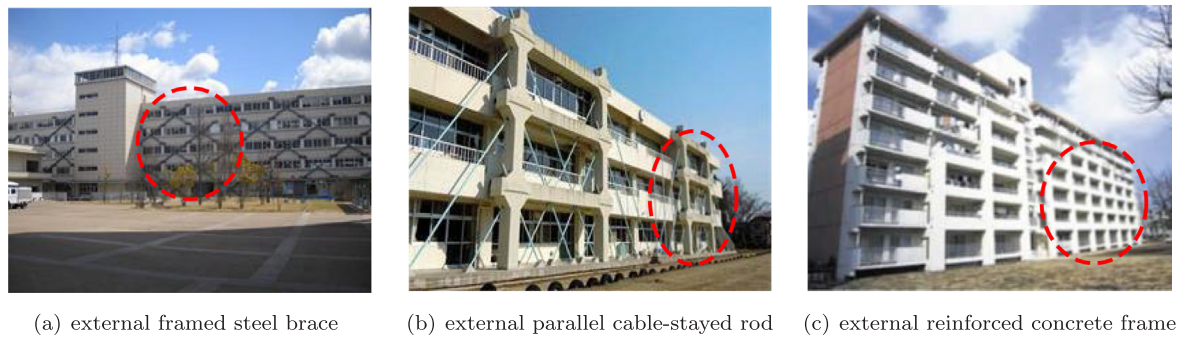
Fig. 1. Typical external sub-structure forms.
