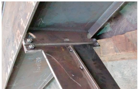
Figure 8 : lower anchorages of the Roboul bridge
