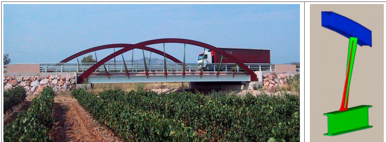
Figure 2 : The Roboul bridge and his welded hangers designed for fatigue
