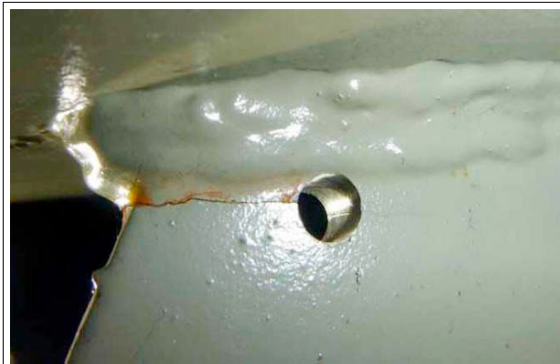
Fig. 23 : Crack at a stiffener attachment at B
