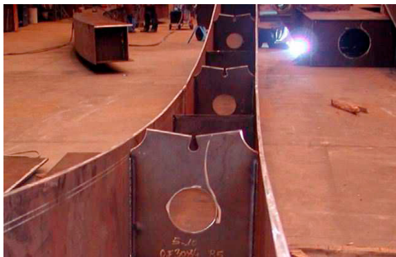
Figure 8 : lower anchorages of the Roboul bridge
