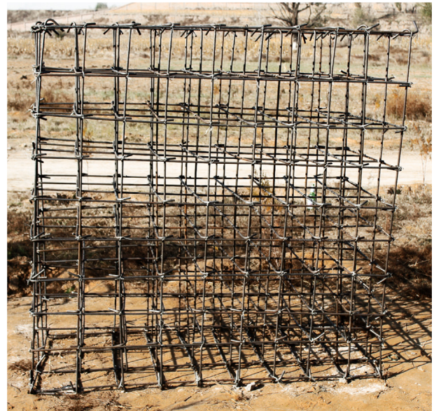
Fig. 6. The layout of the reinforcing bars.
