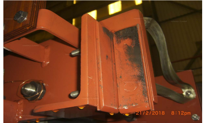
Fig. 4. Overheating signs on the steel wedges between top frame and tank stops
