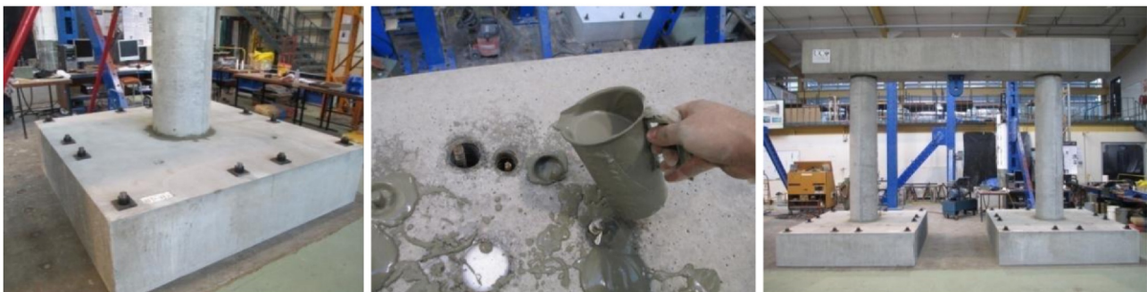
(i) Grouting of Bottom and Top Connections
