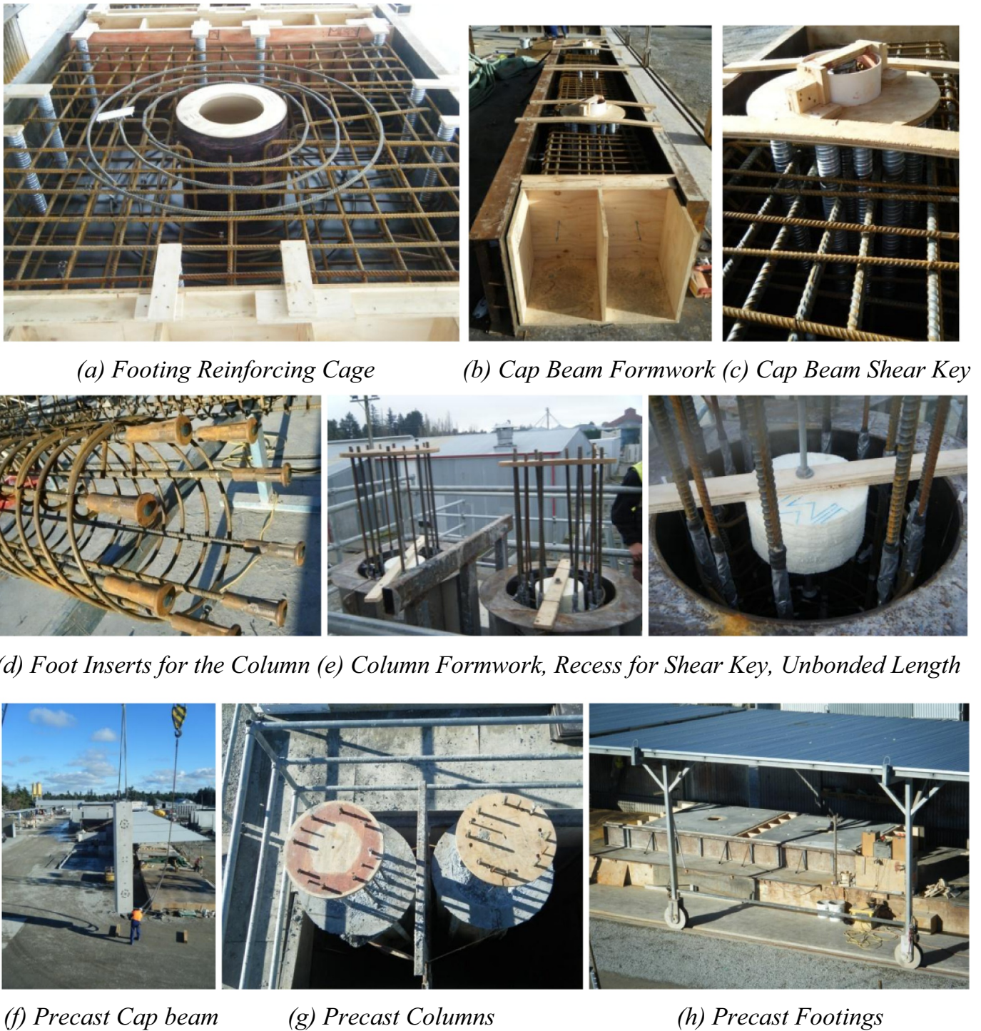
Fig. 8. Photos from construction of precast elements in the bent.
