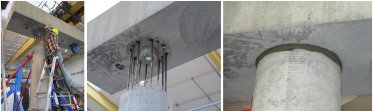
(g) Guiding Column Starter Bars into the Ducts
