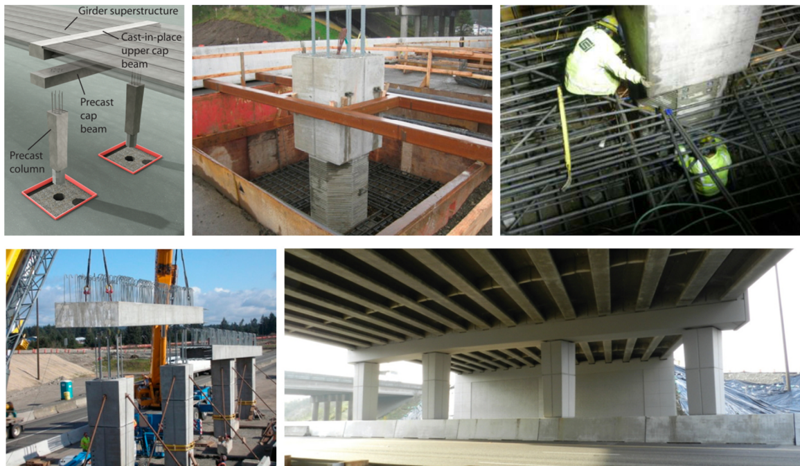
Fig. 20. Precast bent with member socket and grouted duct connections on I-5 in the State of Washington, after Haraldsson et al. [20].
