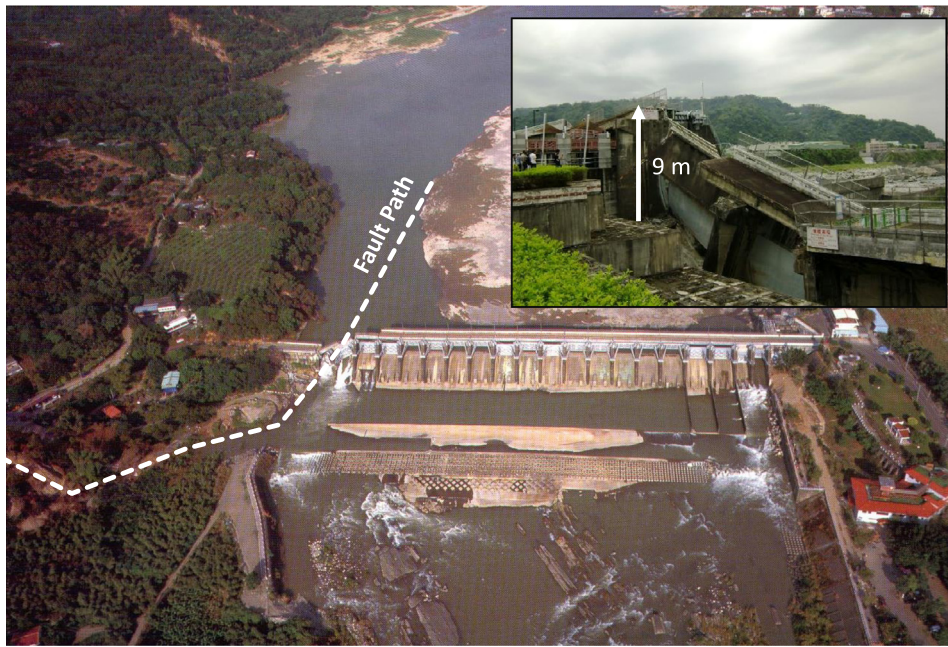
Fig. 1. Damage to the Shih Kang dam due to 9.1 m of upthrust by the Chelungpu fault during the 1999 Chi-Chi earthquake in Taiwan.
