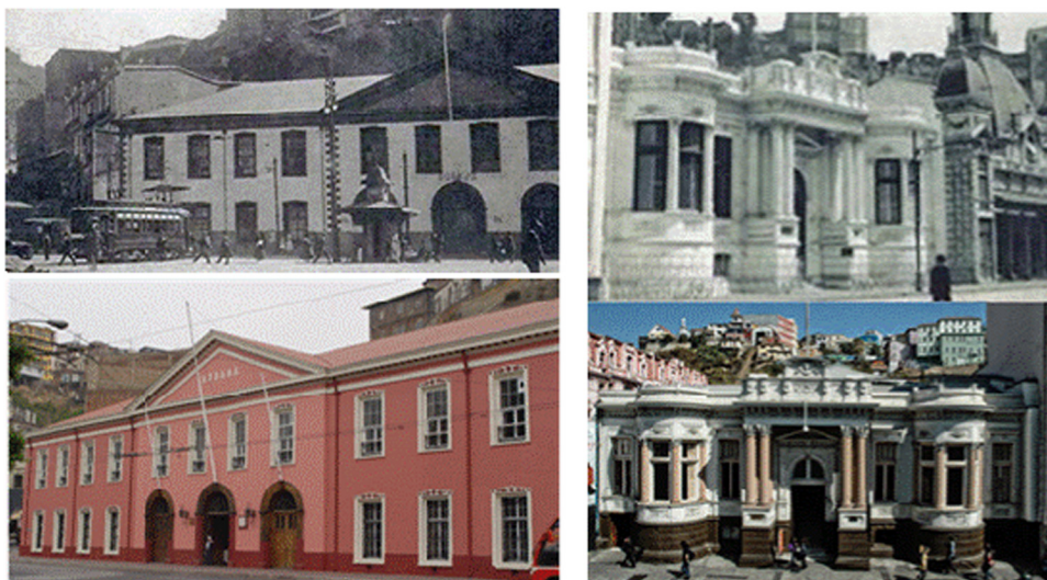
Fig. 5. Aduana (left) and Palacio Lyon (right), examples of buildings founded on bedrock that resulted with minor damages after the 1906 Earthquake, and today are still in usage.
