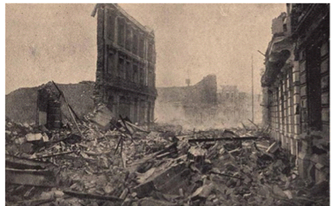
Fig. 3. Total destruction in the area of ground consisting of a sandy soil deposit (intersection of Blanco and Edwards streets).
