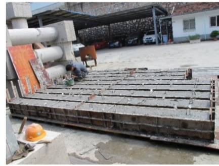
(b) Casting and maintenance of the concrete
