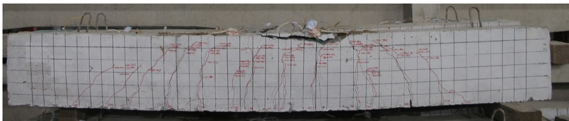
Fig. 8. Failure mode of beam L-3.
