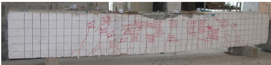
Fig. 9. Failure mode of beam L-4.
