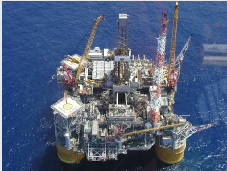
Fig. 23.10 Bird's eye view of the Auger tension leg platform. (Source: Shell, BOEM.)
