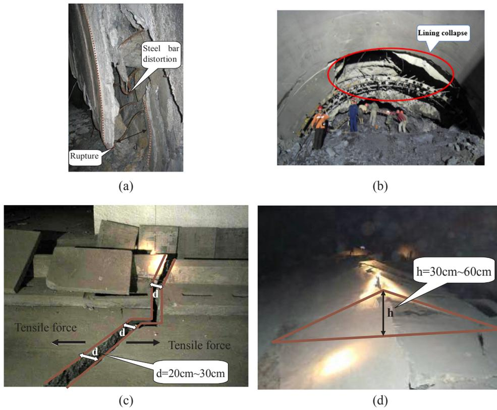
Fig. 1. Damage patterns of tunnel lining in Longxi tunnel. (a) Rupture of Longxi tunnel lining; (b) Tunnel lining collapse; (c) Transverse shear fracture; (d) Longitudinal uplift for pavement.
