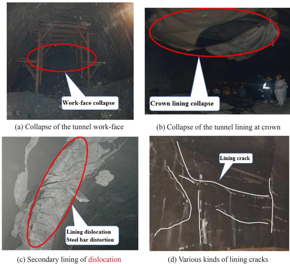
Fig. 2. Lining damage mode of Jiujiaya tunnel. (a) Collapse of the tunnel work-face; (b) Collapse of the tunnel lining at crown; (c) Secondary lining of dislocation; (d) Various kinds of lining cracks.
