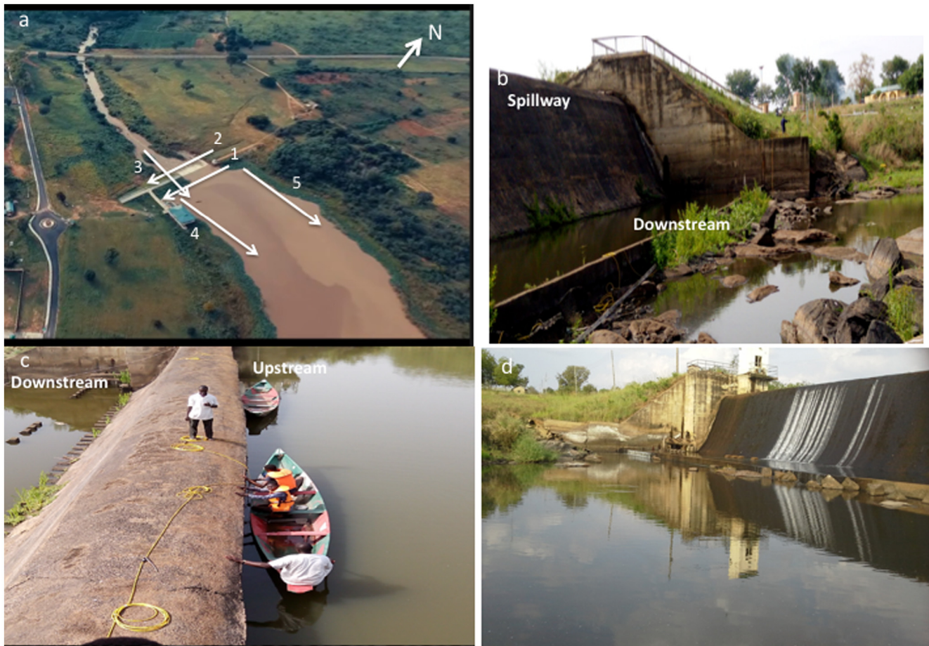
Fig. 2. Aerial and camera photos of the dam environment. (a) Aerial photo showing location of the dam and the 2D resistivity profiles; (b, c, and d) camera photos showing the different sections of the dam.
