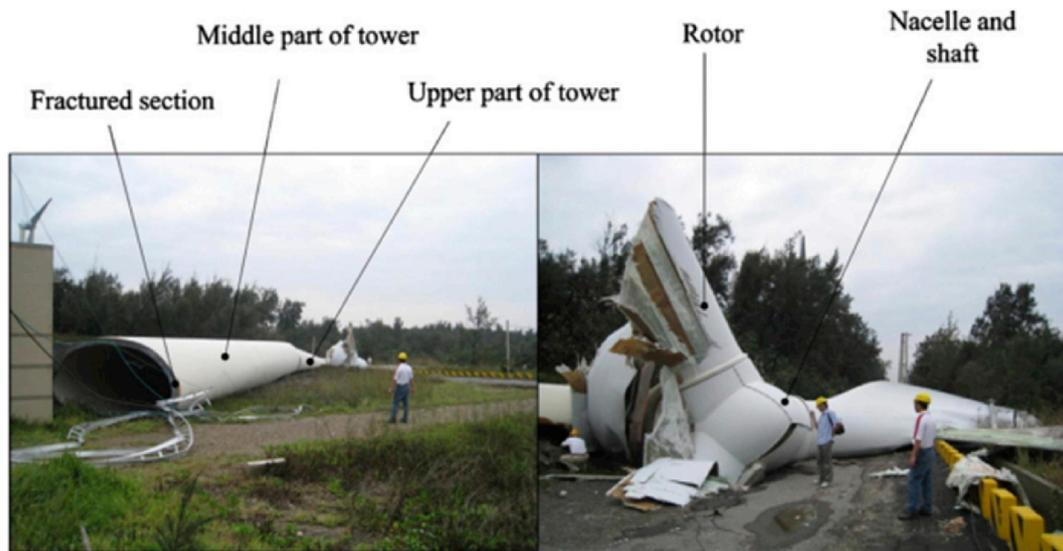
Fig. 4. On site photo of a collapsed wind turbine (after [4]).
