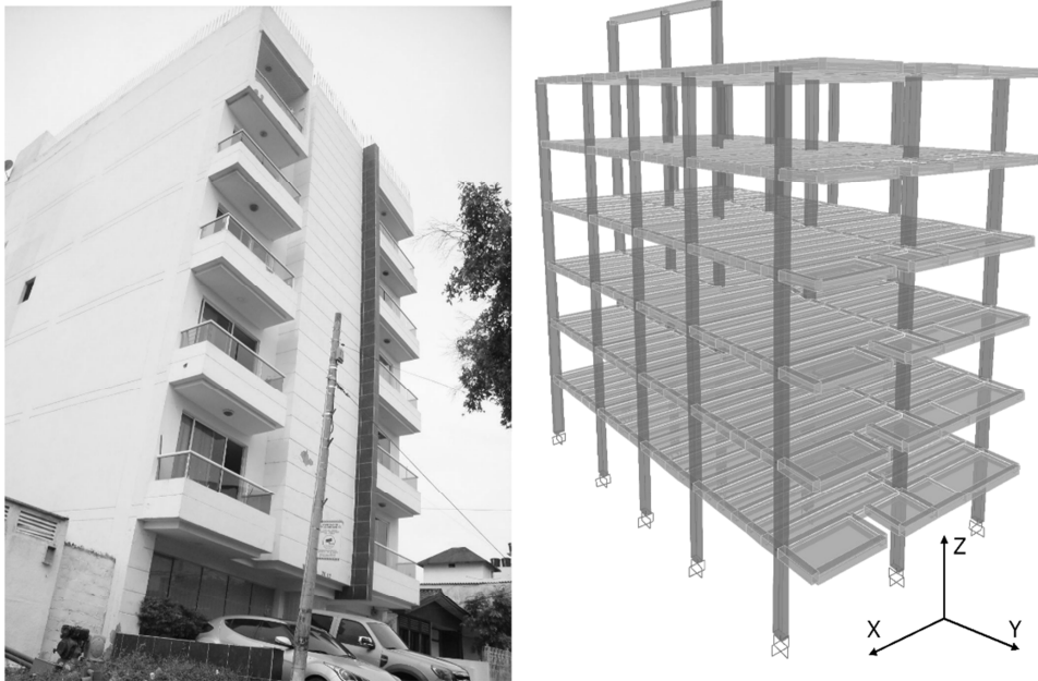
177 178 Figure 5 Left: Existing RC building. Right: Original building Model.
