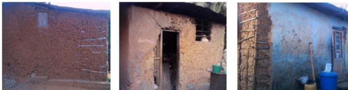
Fig. 2. Typical Wattle and Daub buildings (Source: [8]).
