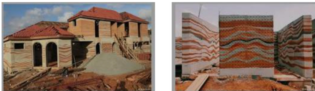
Fig. 4. A typical rammed earth building in Ghana (Source: https://www.dw.com/en/in-ghana ).
