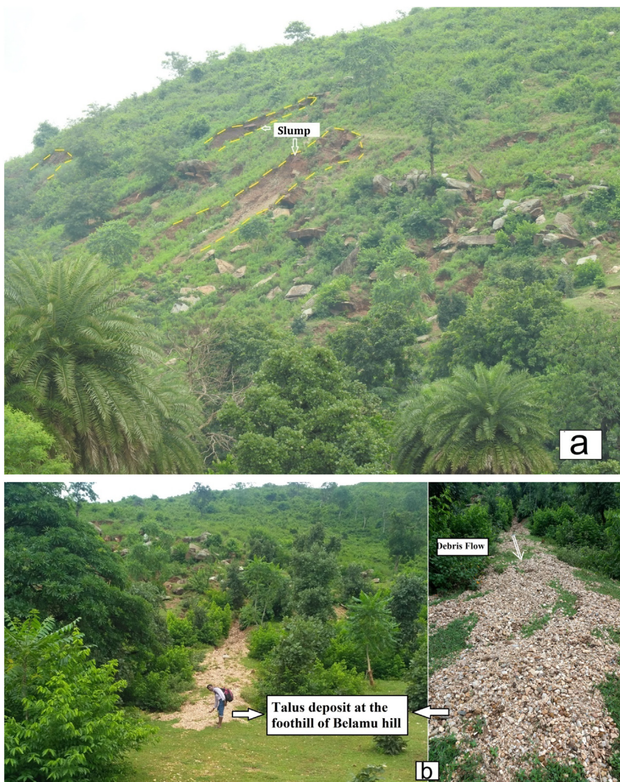
Fig. 3. (a) Heavy rainfall causes unconsolidated red soil to slump, western part of Belamu hill; (b) Deposition of talus at the foothill through debris flow, west part of Belamu hill (southern face).
