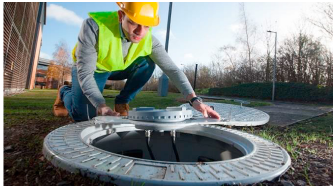
(b) Maintenance-hole cover work as antennas [30].
