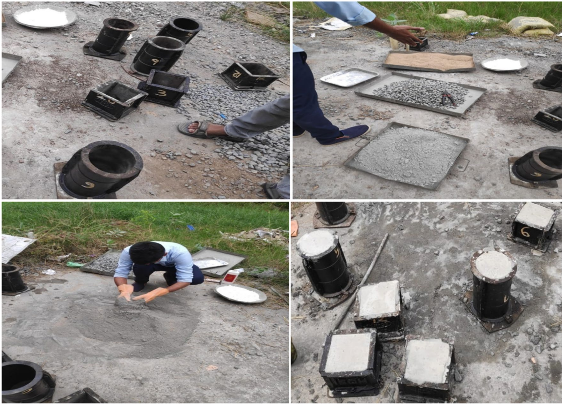
Fig. 9 Placing of concrete in the various specimen
