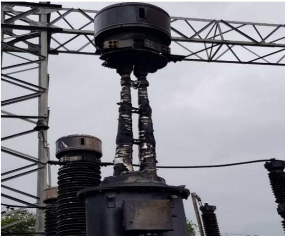
Fig. 10. Kushtia transformer post-CT burst due to transformer fire.
