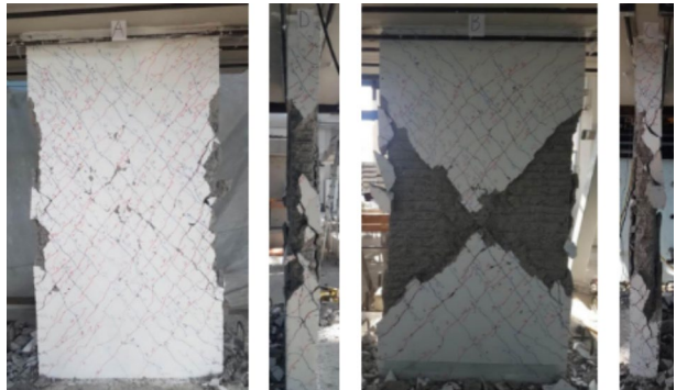
Fig. 18 Crack distributions of P7-2 wall for all faces (A, B, C, D faces)
