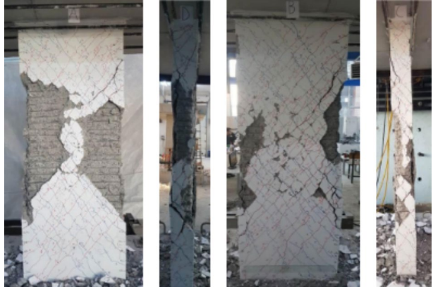
Fig. 16 Crack distributions of P5-2 wall for all faces (A, B, C, D faces)
