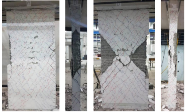
Fig. 17 Crack distributions of P6-2 wall for all faces (A, B, C, D faces)
