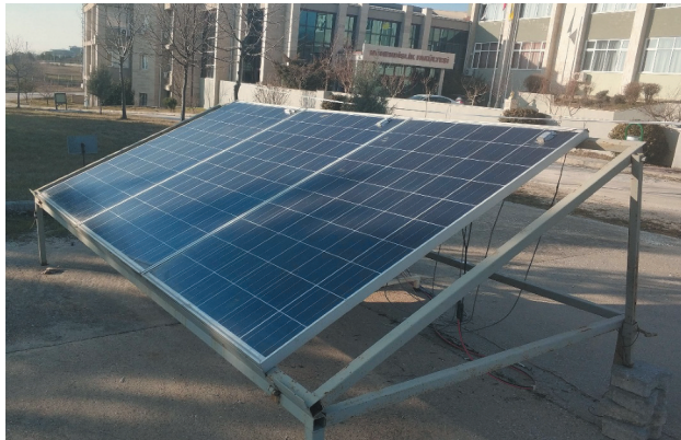
Figure 5. Photovoltaic panel installation.
