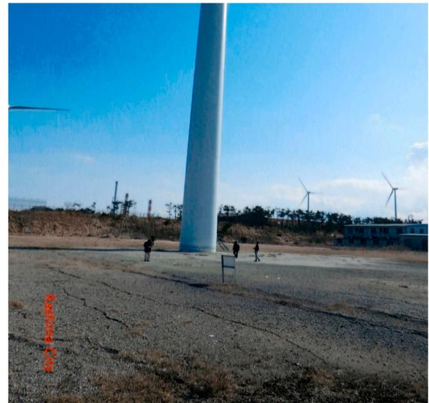
(i) Cracks on ground surface near the tilted turbine indicative of liquefaction induced soil movement
