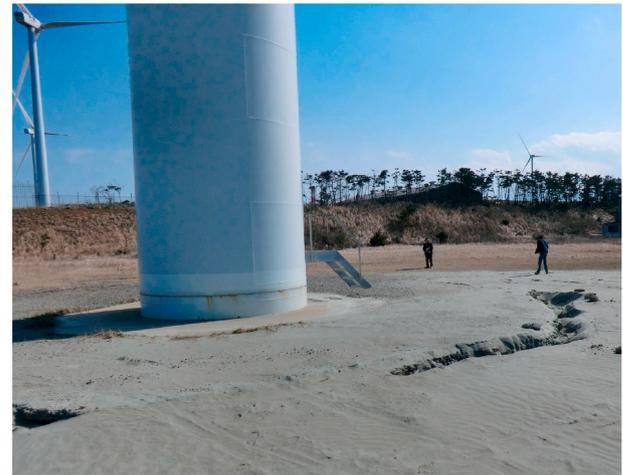
(ii) Soil settlement around the pile cap of the tilted turbine
