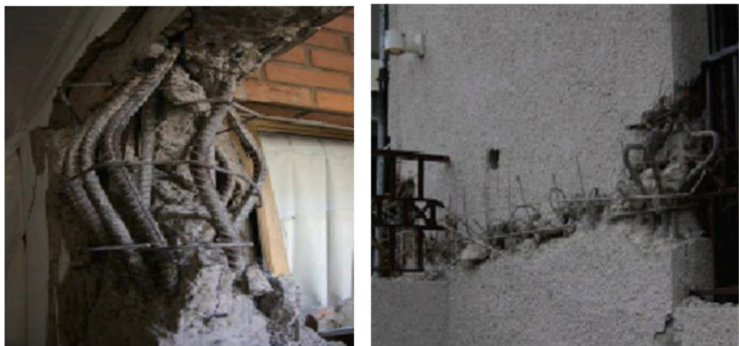
(a) Crushing and rebar local buckling at the end of the wall (b) Concrete crushing accompanied by buckling of the vertical rebars
