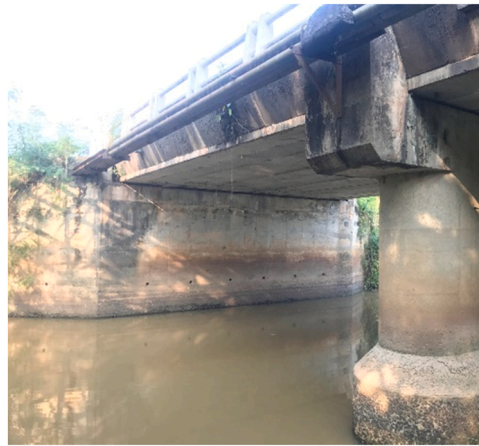
Fig. 4. Veyangoda (B208) Bridge.
