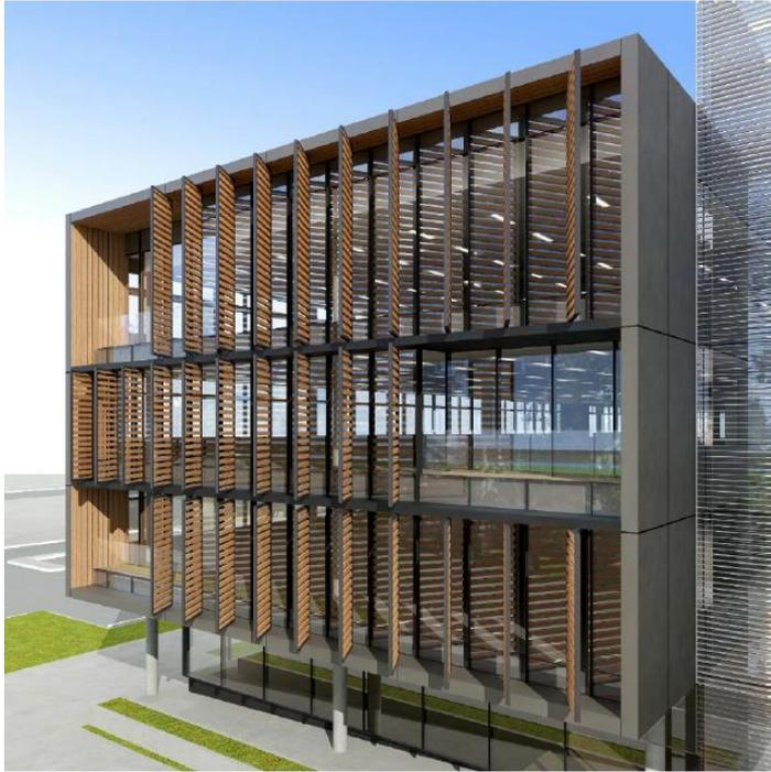
Figure 3-16 Enterprise 1 building east/west timber louvres [79].
