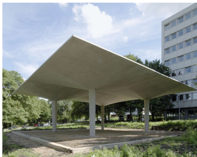
Fig. 1. Roof structure consisting of four large precast TRC shells (photo: bauko 2, RWTH Aachen University)
