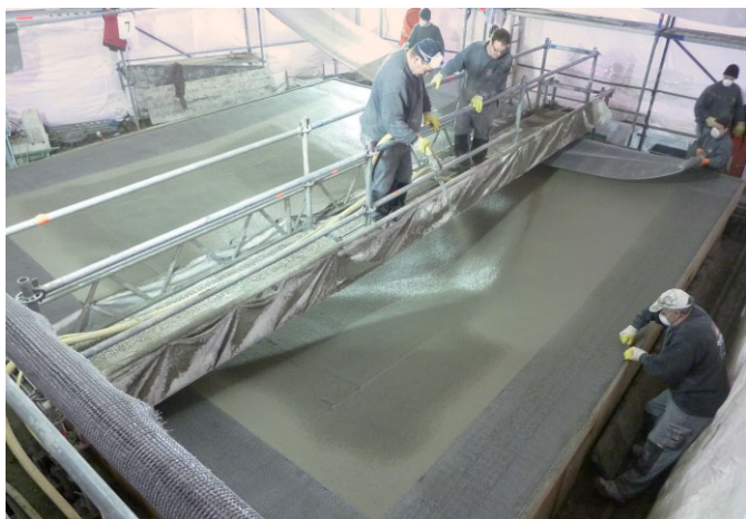
Fig. 13. Production of the TRC shell using shotcrete
