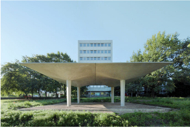
Fig. 15. Loadbearing structure after final adjustment and coupling of the TRC shells (photo: bauko 2, RWTH Aachen University)
