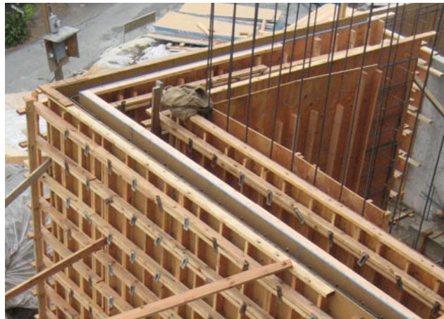
Figure 1: Traditional Wooden Formwork
