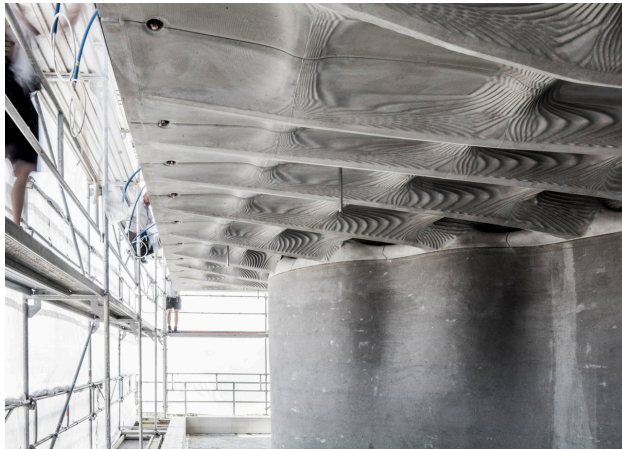
Figure 12: 3D printed floor slab assembly
