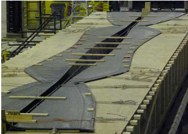
Figure 10: Mark West Full Scale Beam Formwork Bundled up
