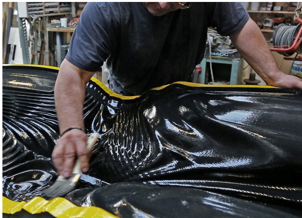
Figure 11: Mold release applied to formwork
