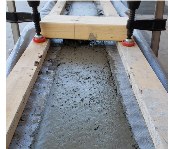
Formwork After Casting
