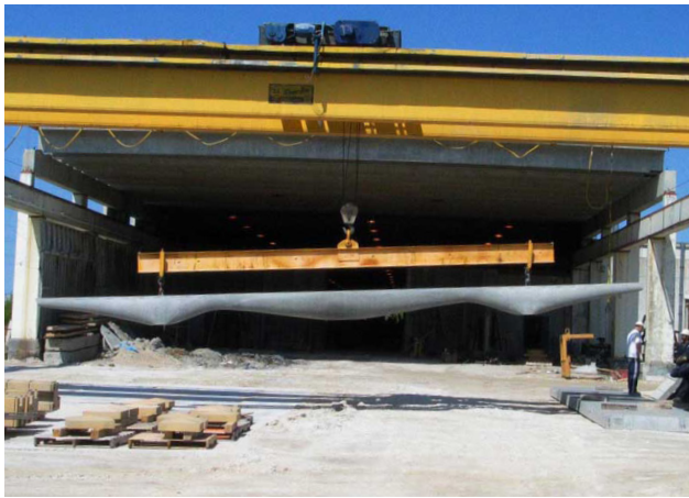
Figure 9: Mark West Full Scale Optimized Flexible Formwork Beam
