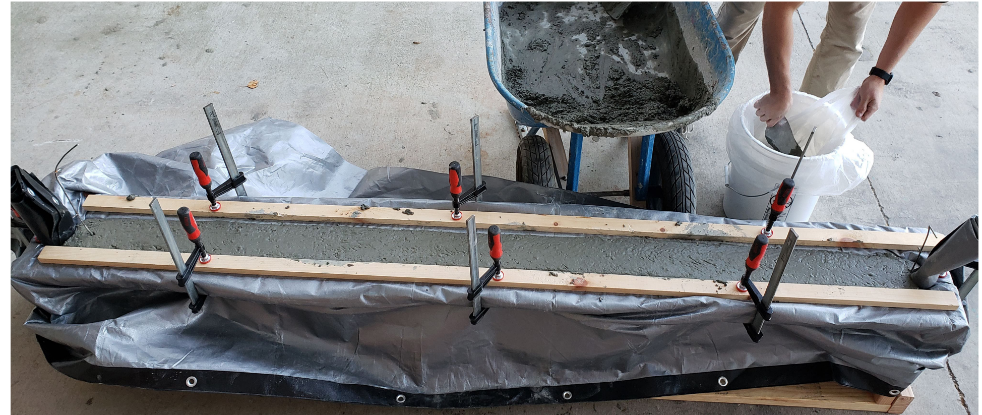
Formwork Before Casting
