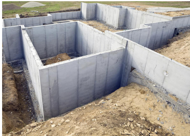
Figure 2: Traditional Wooden Formwork Outcome
