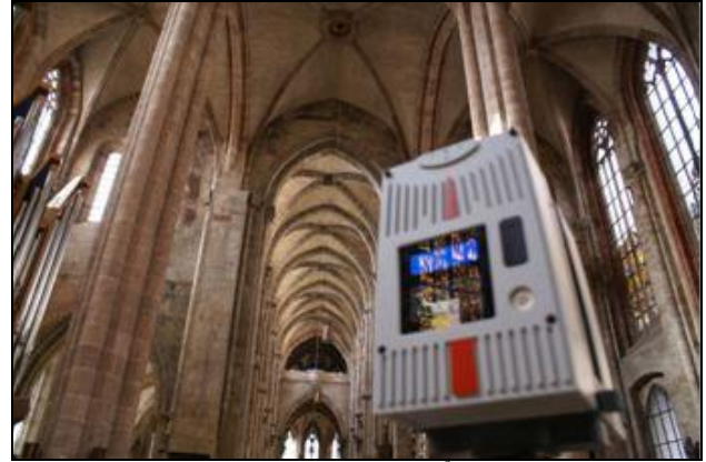
Phase based System used at interior scanning 8
