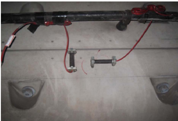
Fig. 10. Strain gauge installed in the segment.
