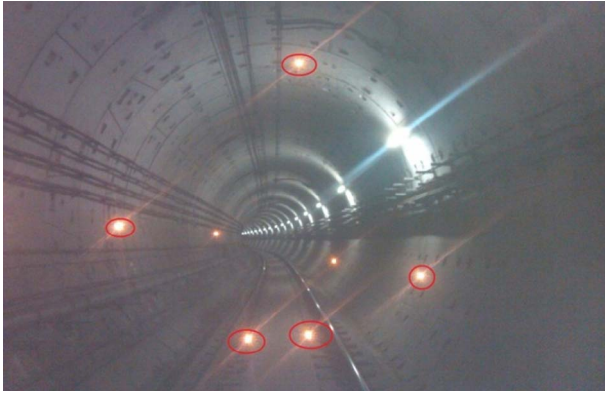
Fig. 8. Measuring points of reflecting prisms.
